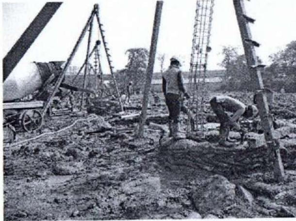
Piling in progress at STP Near WBSETCL, Joka
