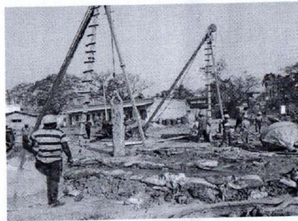
Piling work at STP, Bank Plot, M.G Road
